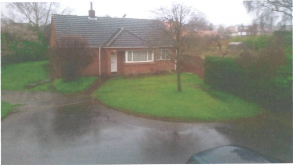
15/02624FUL access route before development
